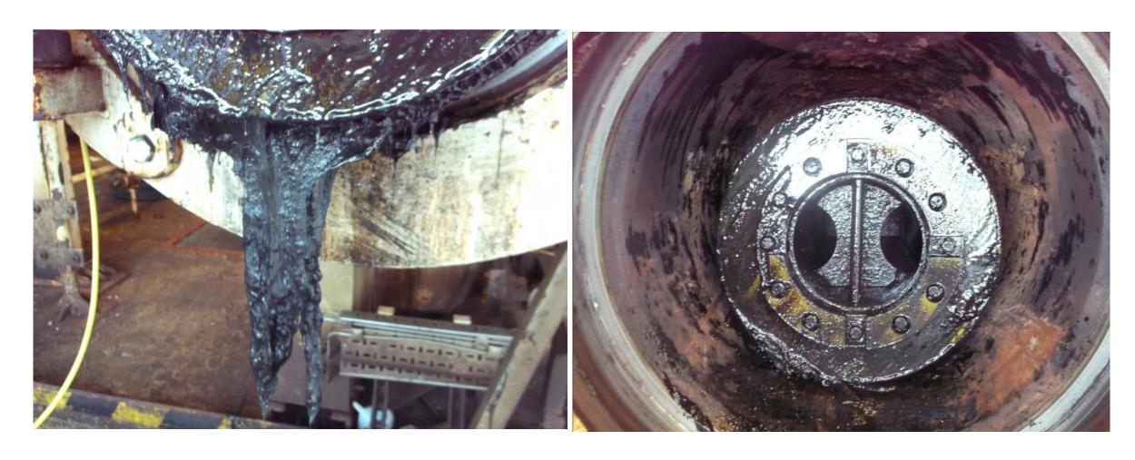
Very heavy and viscous residue recovered by the initial Bi-Di pig runs
