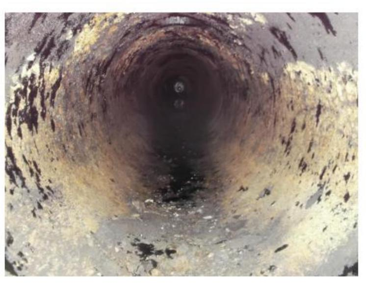
1<sup>st</sup> pig: minimal debris, removed hydrocarbon gas, N2 filled.
