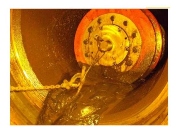
Significant residue still evident after additional pig trains and camera pig run
