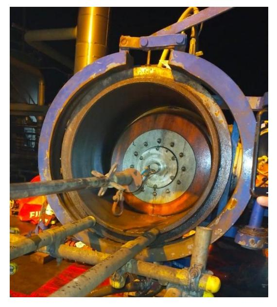
Final pig run, minimal residue and debris
